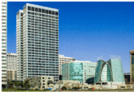
1 Kaiser Plaza – Existing Building
