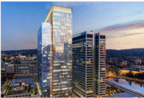
2 Kaiser Plaza (Beacon Tower), Oakland, CA
