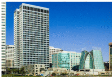
1 Kaiser Plaza – Existing Building
