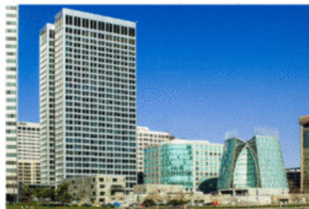
1 Kaiser Plaza – Existing Building
