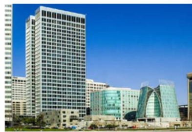
1 Kaiser Plaza – Existing Building
