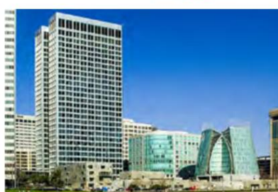
1 Kaiser Plaza – Existing Building
